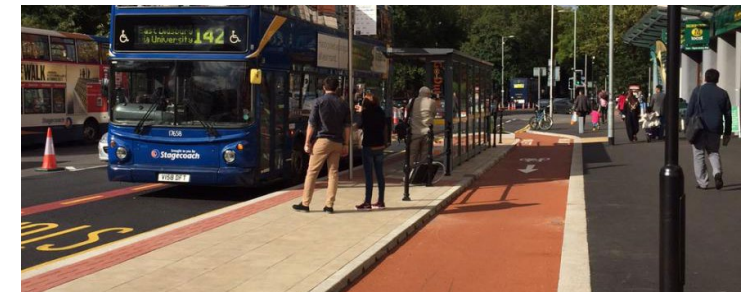
Image 5.2.5. Pavement Improvements, Manchester, UK
